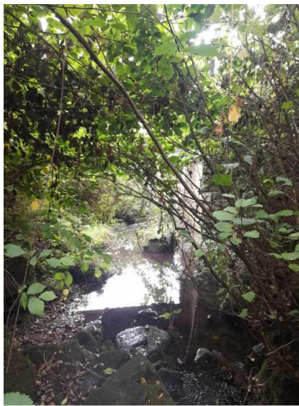
Looking into one of the inaccessible areas
